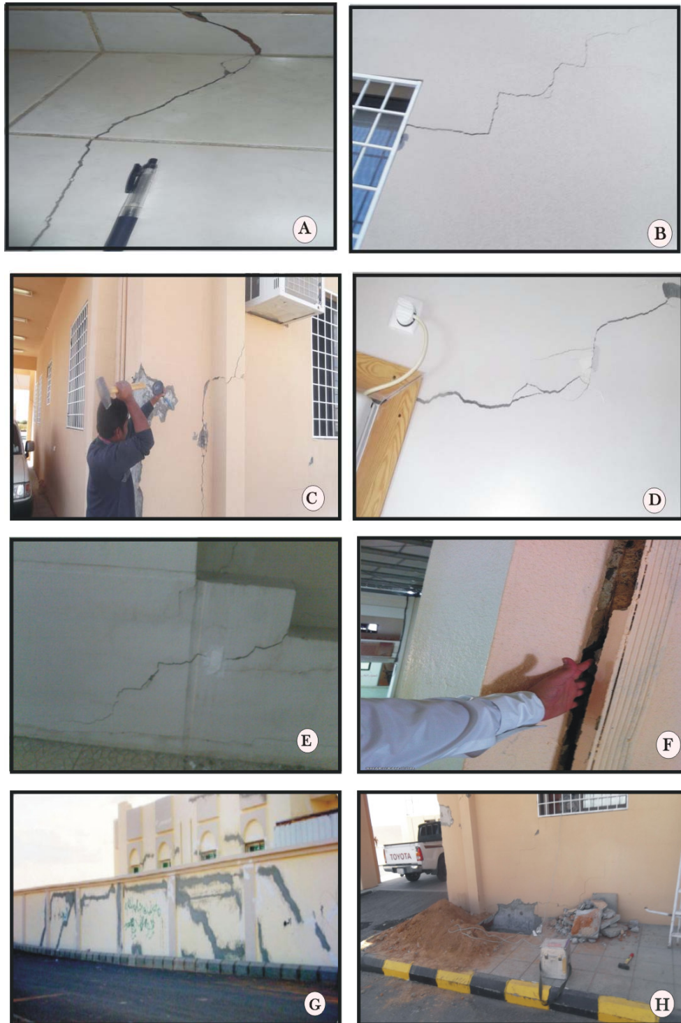
Fig. (4): Damage to the buildings has been caused mainly by differential heave of the foundation sub-soils, A; B; C and D, the cracks are typical expansive soil cracks being wide at the top and getting narrower at the bottom of the wall. G and D cracking of reinforced concrete gates, columns and ground beams at different sites of study area.
